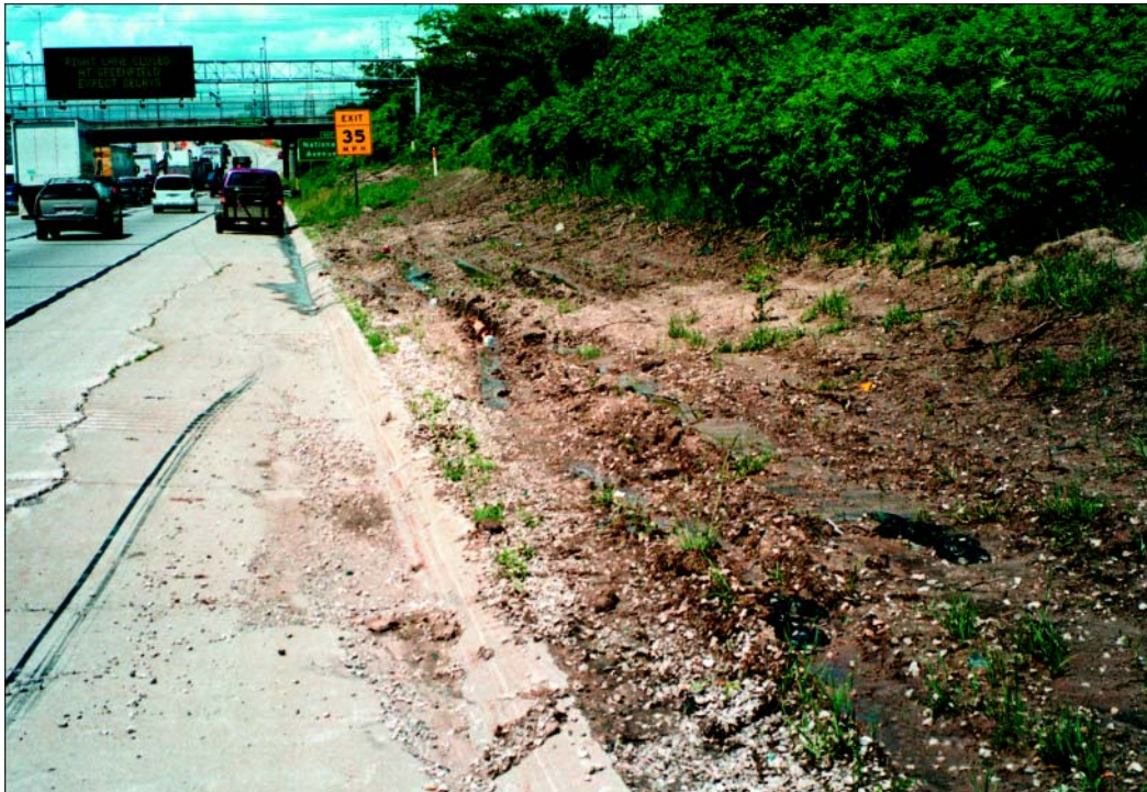
Figure 3. Example of dirt and gravel from utility construction on highway shoulder.
